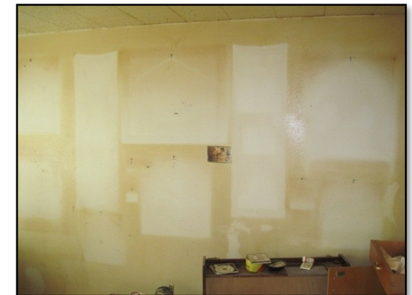
A home where family members smoked inside. This shows the wall once pictures were removed. Nicotine and smoke chemicals stay on the wall.
